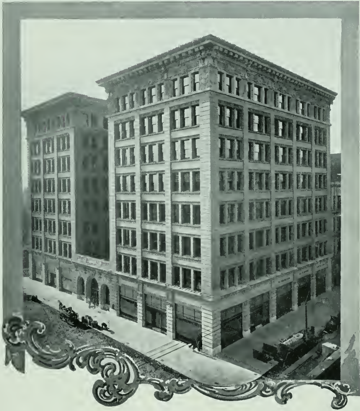
RIALTO BUILDING. Cor. Mission and New Montgomery Streets.
